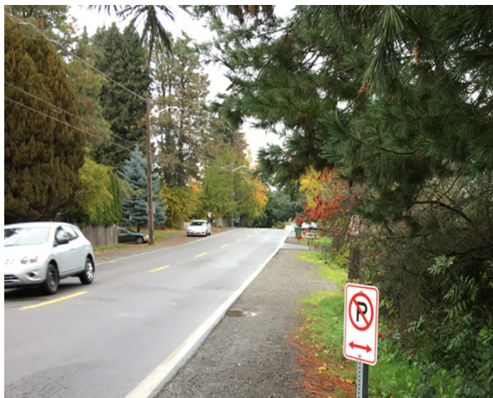
Existing gravel shoulder where we'll build the new sidewalk
